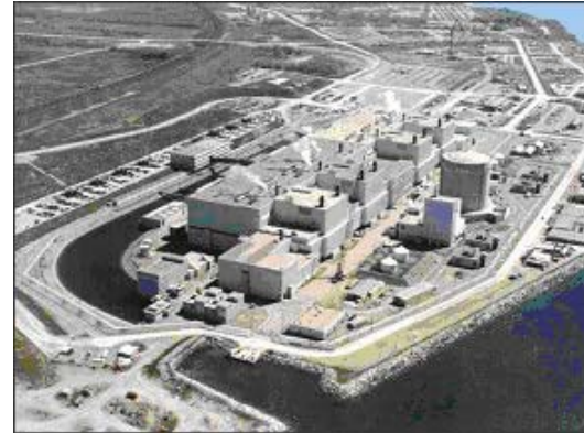
Darlington Nuclear Generating Station
